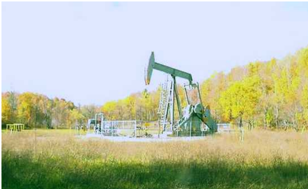
Typical Michigan Oil Well
