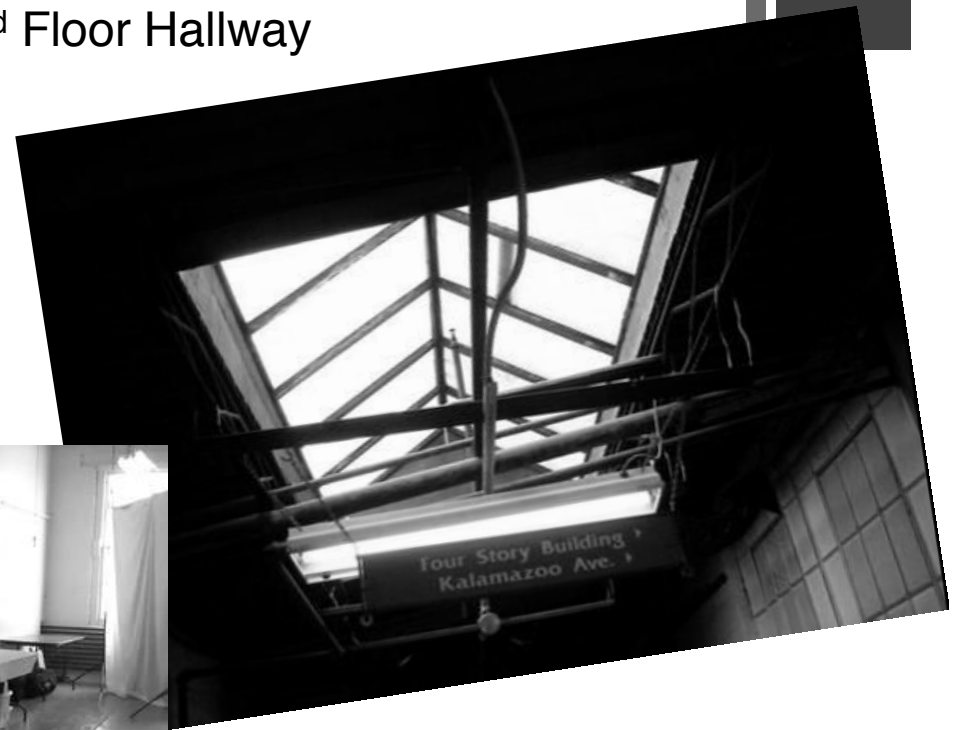
Skylight in North Building
