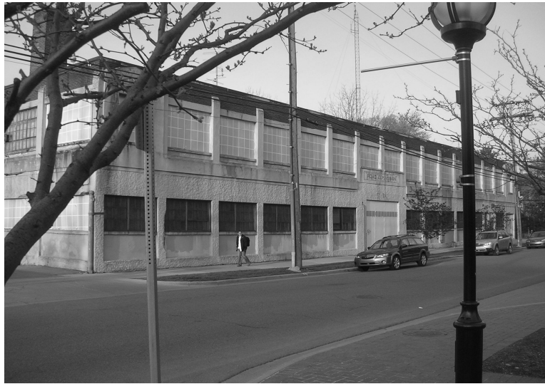
Existing buildings masonry/concrete wall construction
