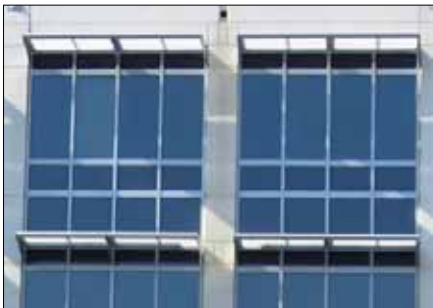
Exterior light shelves placed above windows reduce solar gain during the summer months.
