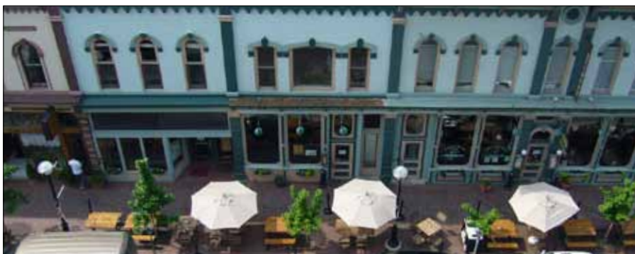
Maintain the traditional window spacing alignment patterns of upper floor in Main Street.
