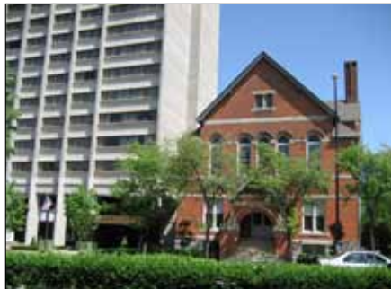
Most buildings in East Huron are set back from the sidewalk.
