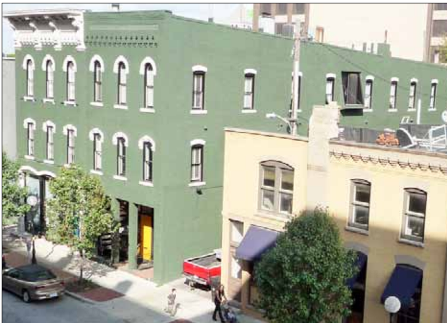
Traditional commercial buildings in downtown Ann Arbor share similar features while also being distinctive. Masonry is the most commonly used material, and upper story windows establish a consistent rhythm that visually links storefronts.
