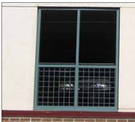
Architectural screens above the first floor of a parking structure help minimize the visual impact of parked cars and promote a pedestrian friendly street edge adjacent to the structure .
