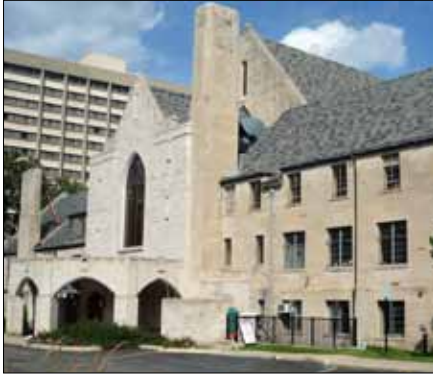
The First United Methodist Church stands out as a landmark building, providing a unique accent in the East Huron Character District.
