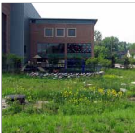
The storm water retention basin at the Ann Arbor YMCA provides an example of a natural storm water system and retention basin.
