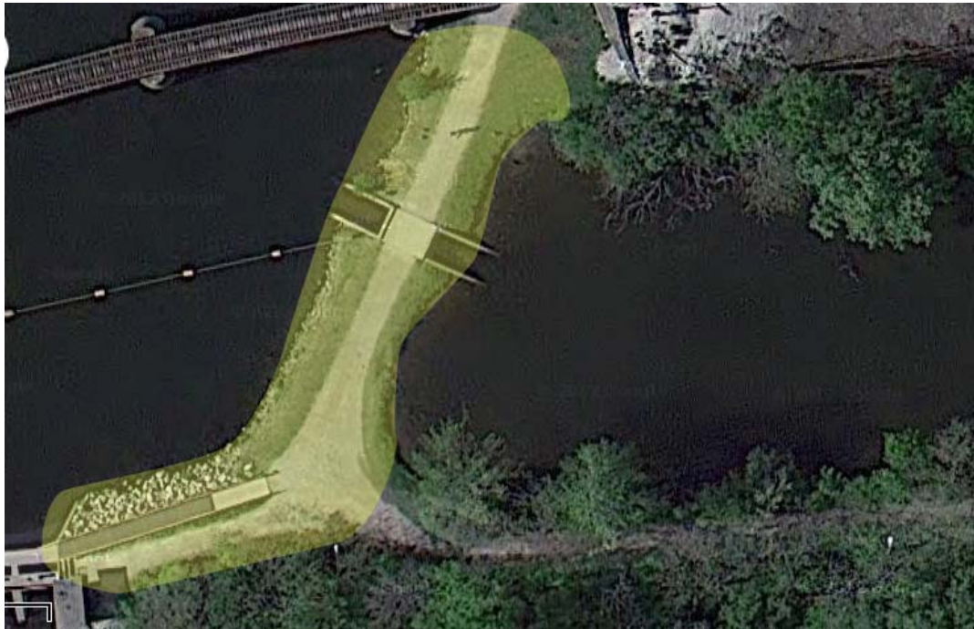
Ariel photo depicting the State regulated embankment. Photo taken before the Cascades were built.
