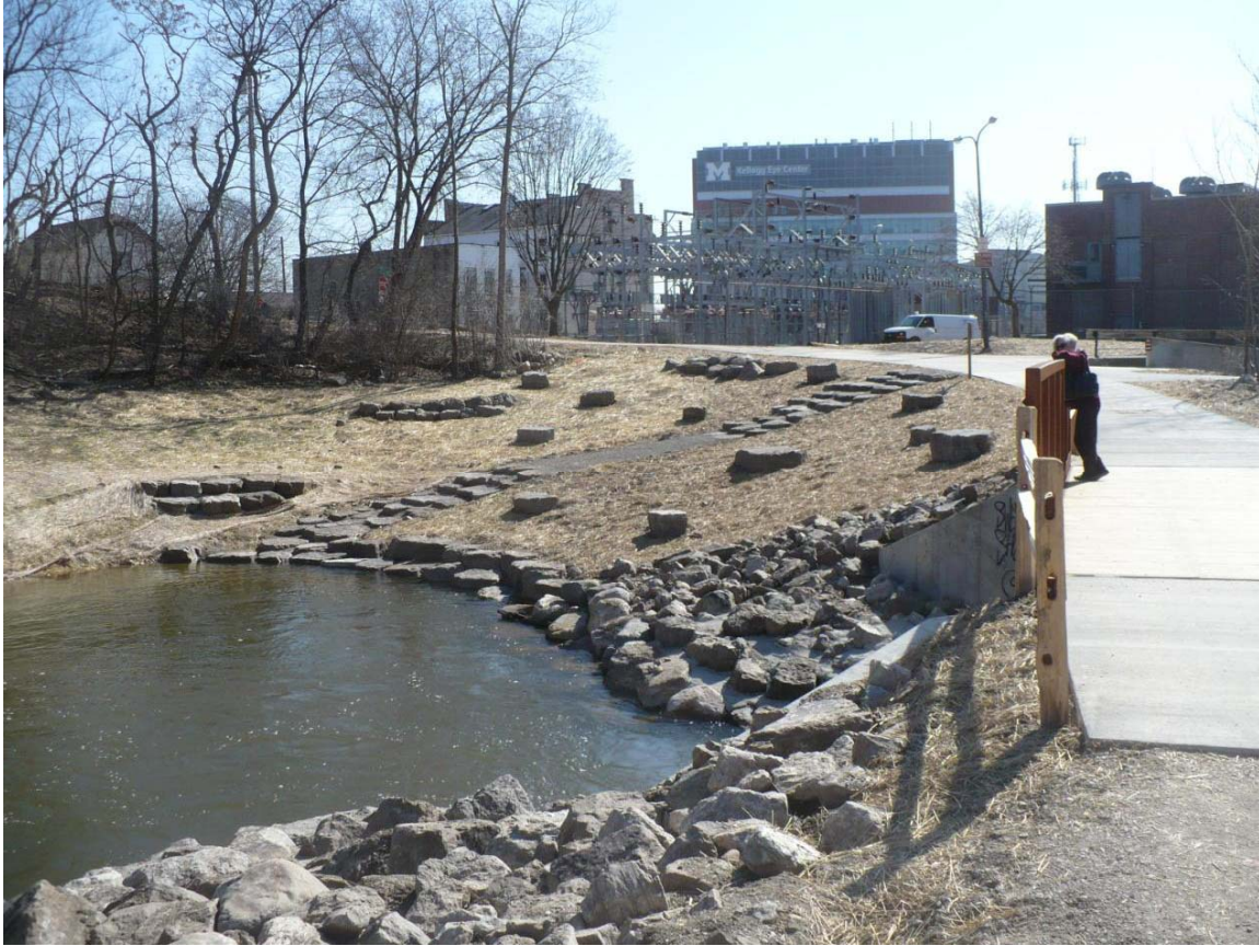
Riverbank at Cascade's toe and Exit Bridge, facing east
