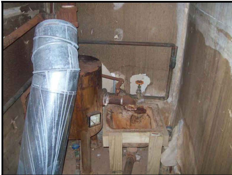
PHOTOGRAPH NO. 13: FORMER DRY CLEANERS LOCATION OF FORMER DRY CLEANING MACHINE
