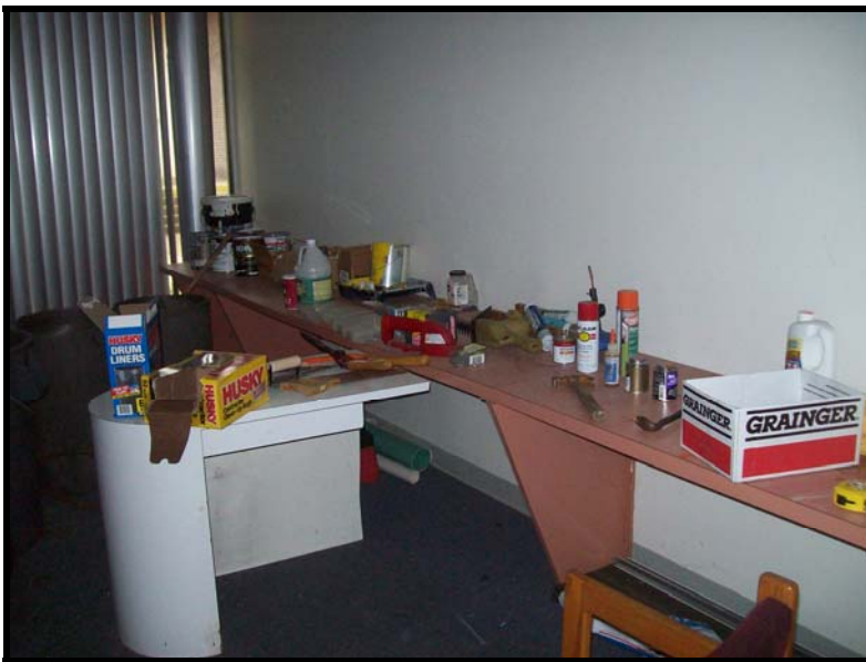
PHOTOGRAPH NO. 7: SUBJECT PROPERTY FORMER STUDIO 13 SALON AND SPA – 5216 PACKARD STREET (NOTE MOLD ON BACK WALL)
