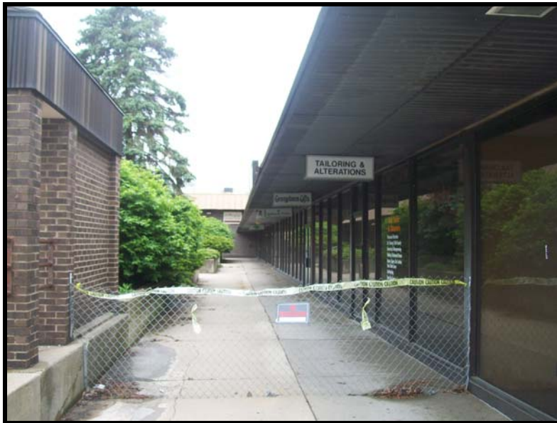
PHOTOGRAPH NO. 3: SUBJECT PROPERTY – FORMER OFFICE BUILDING TYPICAL OFFICE AREA
