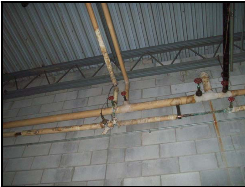
PHOTOGRAPH NO. 19: FORMER KROGER'S FORMER SHIPPING AND RECEIVING AREA
