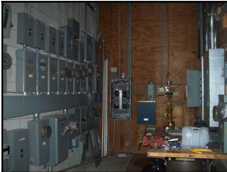
PHOTOGRAPH NO. SUBJECT PROPERTY FORMER ANTHONY'S PIZZA – 2520 PACKARD STREET
