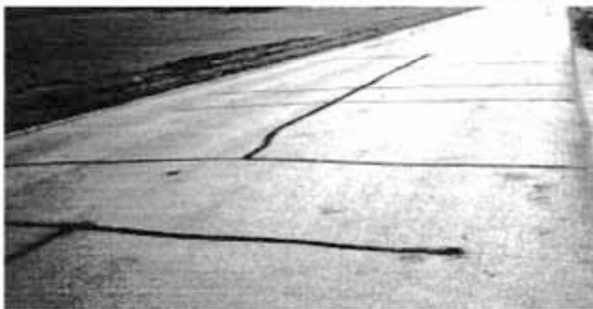
▼ Open crack, 1/2" wide; adjoining pavement sound
