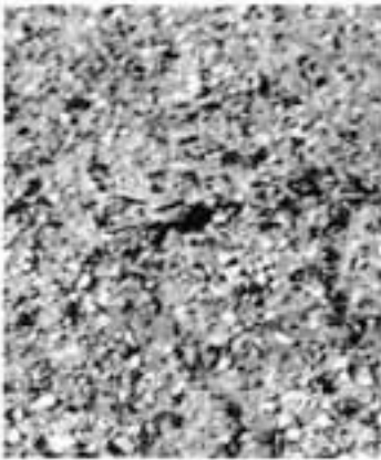
Severe raveling with ▼ extreme loss of aggregate
