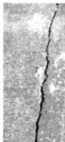
▼ Open crack, 1/2" wide; adjoining pavement sound
