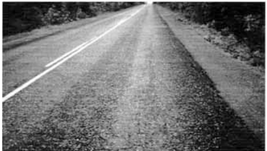
► Moderate to severe raveling in wheel paths.
