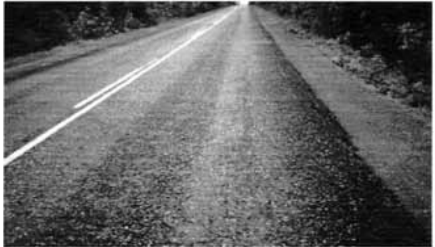
► Moderate to severe raveling in wheel paths.
