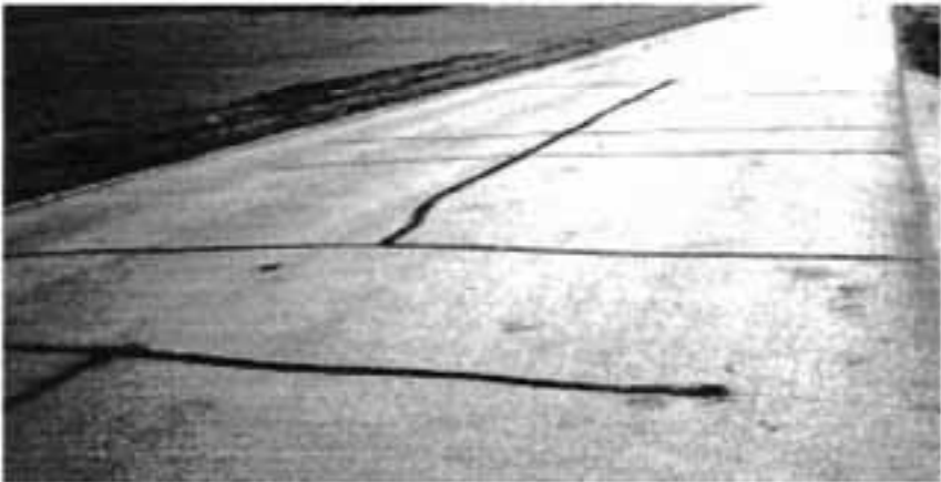
Open crack, 1/2" wide; adjoining pavement sound
