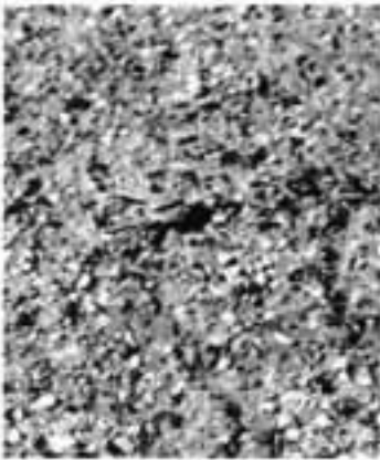
Severe raveling with ▼ extreme loss of aggregate
