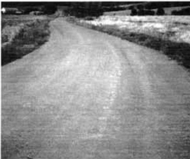
▲ New cold mix surface.
