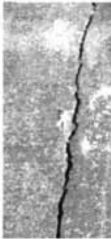
Open crack, 1/2" wide; adjoining pavement sound
