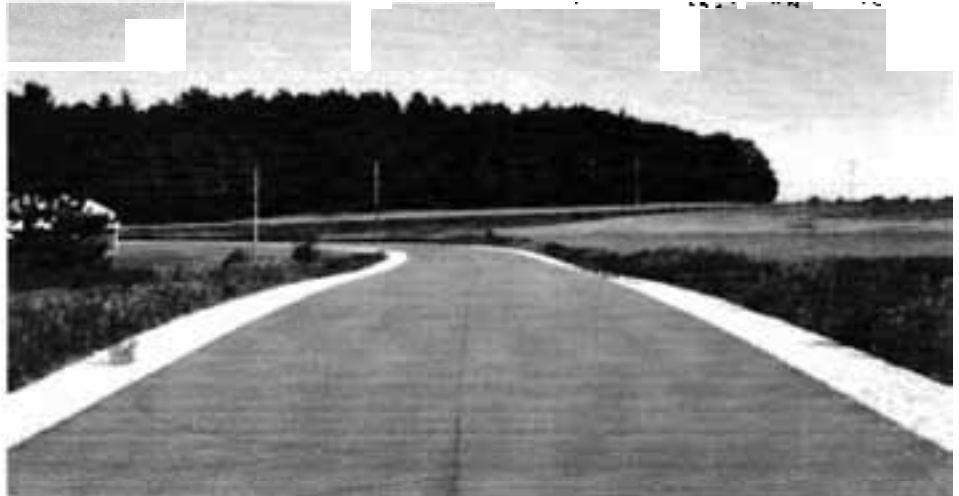
▶ RATING 10 New construction.
