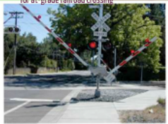
6 Auto/pedestrian/bike gate for at-grade railroad crossing
