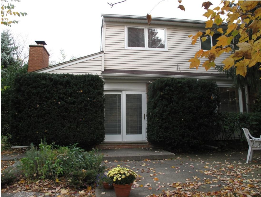
Note: Existing rear door and gable roofline to be matched and continued for porch
